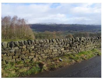
Dry stone walls (like the one shown on the left) are a feature of the British Countryside. There are estimated to be over 5,000 miles of these mortar-less walls in the Yorkshire Dales alone, some dating back over 600 years. Typically they are a "double" wall and are constructed by placing two rows of large stones and filling the gap with smaller stones and rubble.
